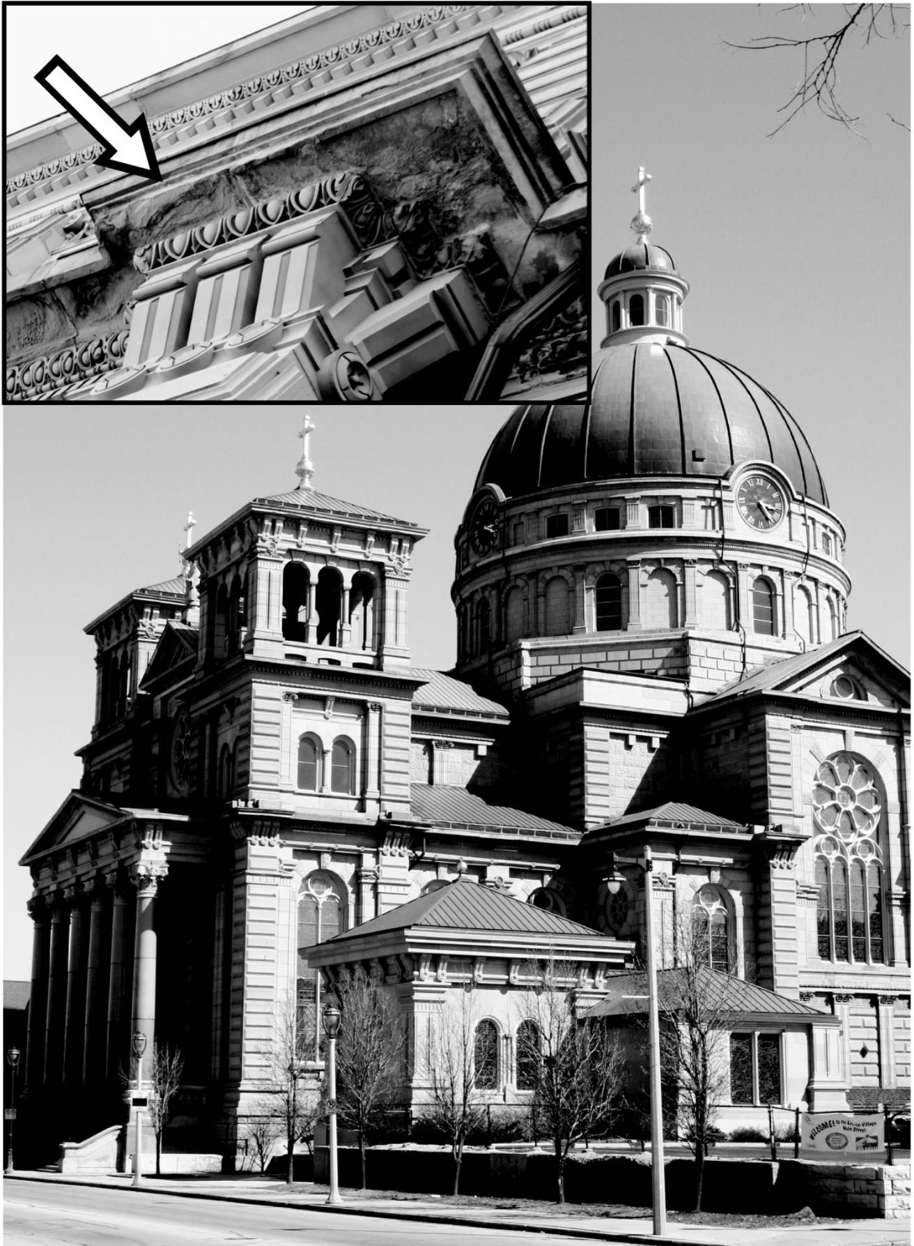
**FIGURE 6.** Photograph of St. Josaphat Basilica constructed with stone from the Buena Vista Member. April, 2008 photo. Inset photograph showing weathering on the underside of the overhang (arrow). April, 2008 photo.
